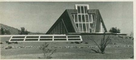
DESIGNED TO FIT its mountain and desert surroundings, the *House of Dreams'* unique features include solar collectors for heat and hot water supply and high earth banking against both heat and cold. (The Ahwatukee House has other non-electronic unique features. For example, there is not a square room in the house.)
